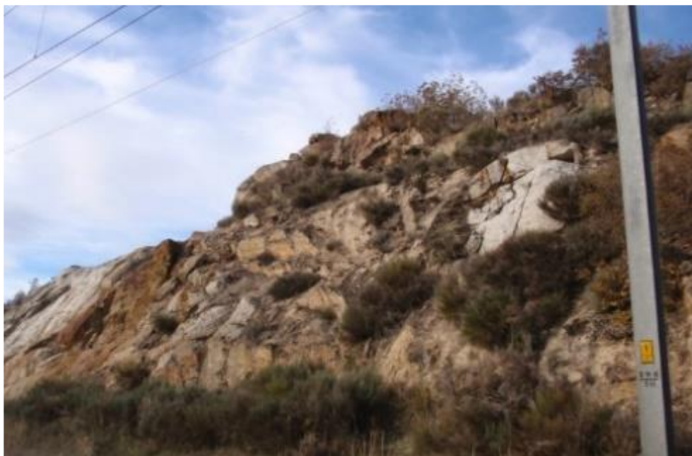
Figure 3.3: Photo of the slope (Costa, 2019).
